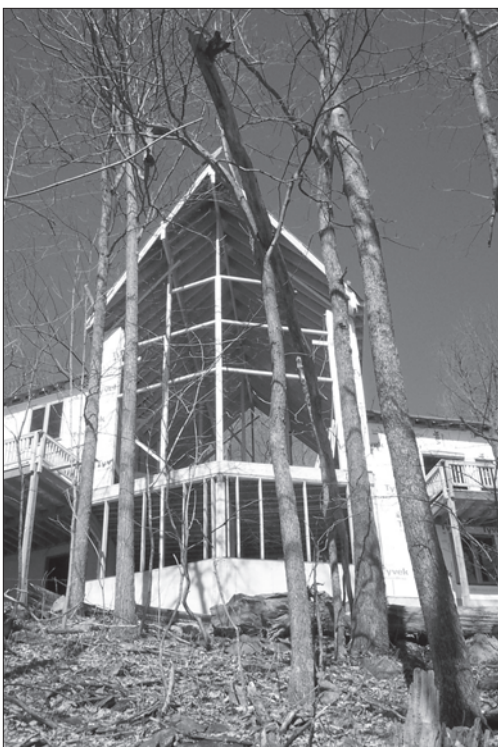
Steve Crandall (top right) is owner of design-build firm Tectonics II, an independent dealer of Lindal Cedar Homes. This mountain contemporary in Wintergreen (left) is an example of the company's green construction (Details page 10). Crandall employs roughly 20 employees in the office and on the field (opposite, bottom).
